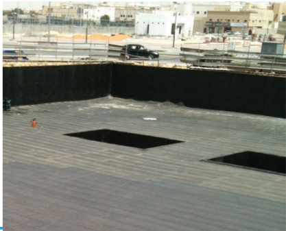
Roof Sheeting EPDM
